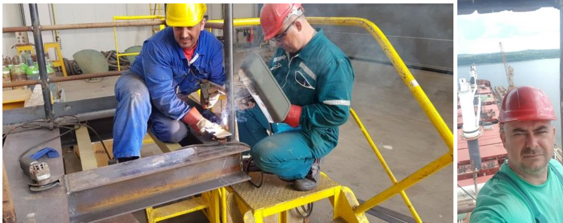
Figure 5. Pictures from ship repair activities of structures in MTG Dolphin
